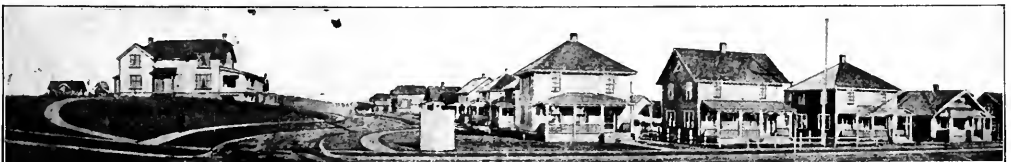
On the left is Director's House, facing Cambridge A ve. Houses in front, on Seventh Street, are occupied by Superintendents, the Mayor, and other dignitaries.
